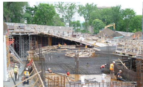
June 2017 / Laying of reinforcement in the agora roof concrete slab
