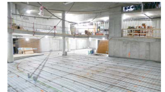
December 2017 / Preparatory work on the agora's slab on grade
