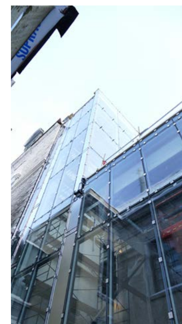
January 2017 / Curtain wall of the Parliament Building's elevator shaft
