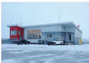
Renovated terminal building in Tasiujaq. Important terminal building upgrading and renovation work has been completed in recent years at various community airports.
