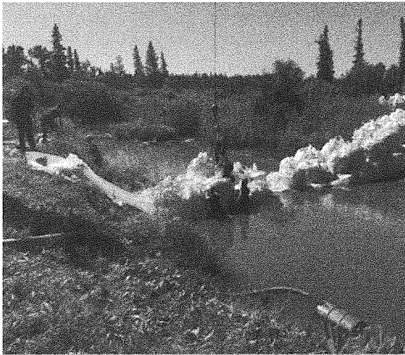
Crews in Prince Albert, Sask., have deployed pipes and a pumping system Little Red River Park to draw water from the Spruce River to supply the city water treatment plant. (CBC)
