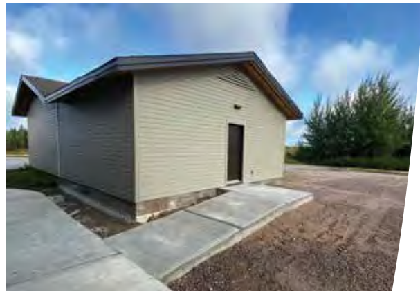
Justice Wemindji warehouse expansion
