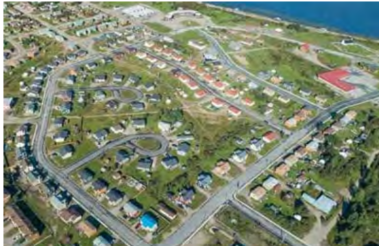
Waskaganish Pavement Catch-up Program in Existing Streets
