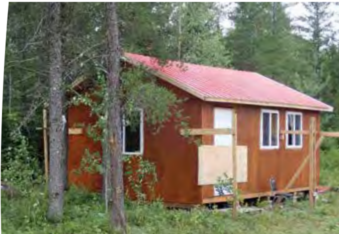
Spot Check on Mistissini cabin renovation, August 2020 (Talleyman: Stanley Mianscum)
