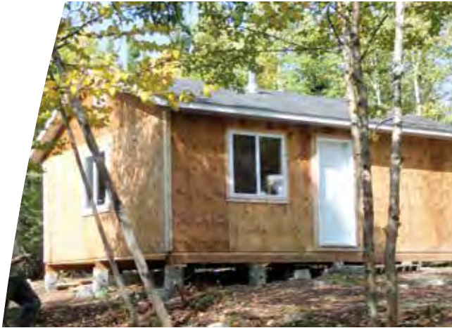
Spot check on Nemaska cabin construction, September 2020 (Talleyman: Billy James Jolly)
