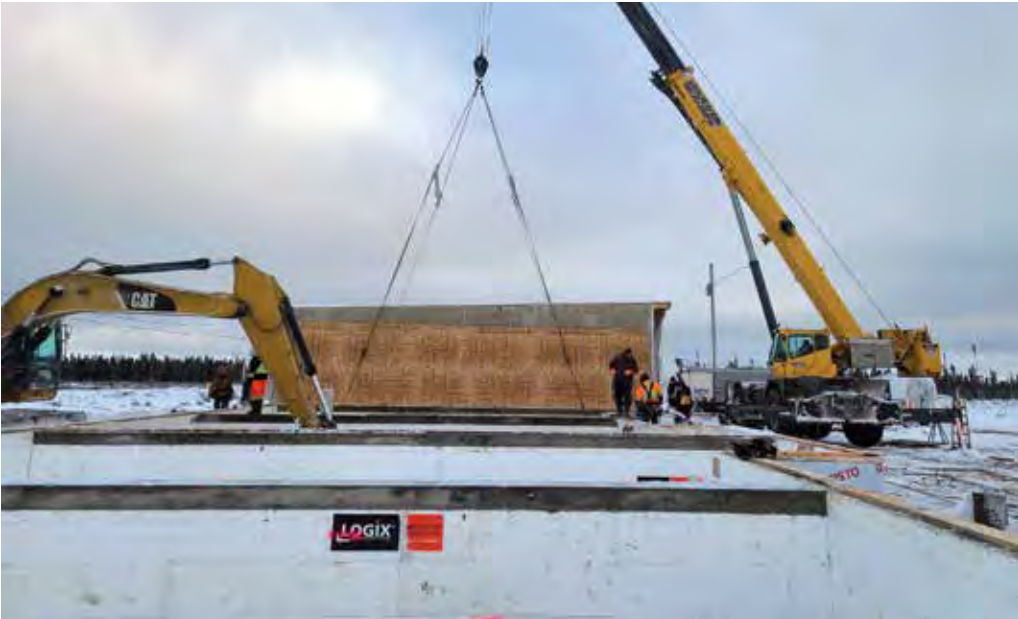
Modular units being installed on the foundation
