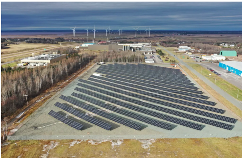
Figure 5 : Community Solar Garden, Amherst Nouvelle-Écosse (Nova Scotia Power)
