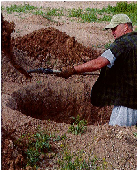
Figure 4 : Excavation manuelle
